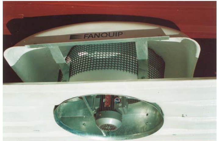
Underside view showing hood supports and birdmesh.
