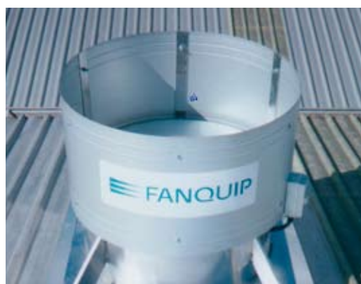
Fanquip VDR Fan clearly showing the windband. The butterfly dampers are just visible in the closed position as the fan is not in operation.
