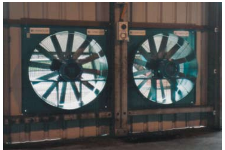
Inlet Side → Showing mounting off purlins.
