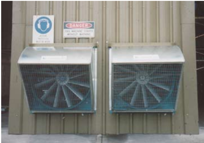
Inlet Side → Showing mounting off purlins.
